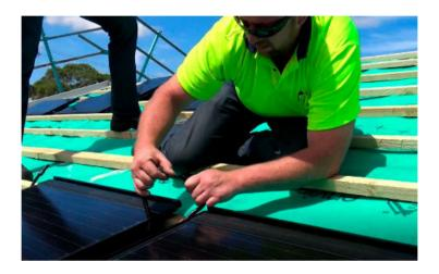
The AC wire must remain in the in the wire containment box of the first and last solar unit of each row. The lead connector and the same made in situ, are fitted in flexible and solid HD conduits between the isolator and the first and last modules to complete the circuit.
